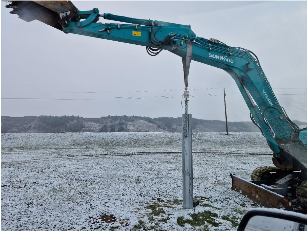
Fig. 10. Metallic profile during vertical tests
