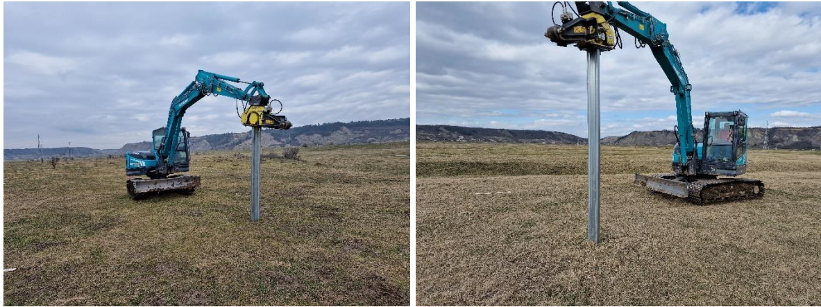
Fig. 5. The ramming process of the metallic profiles
